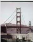
San Francisco, California Architectural photographs A-5 = G.G. bridge from south end.
